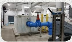
for corrosion control. This process utilizes air stripping rather than the injection of sodium hydroxide to raise the water's naturally lower pH. The system also reduces the cost of water produced at the well – a nice side benefit!
