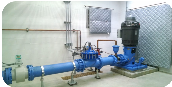
Well 5 Main Pump Room
