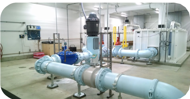
Well 5 Lowry Tanks and Booster Pump
