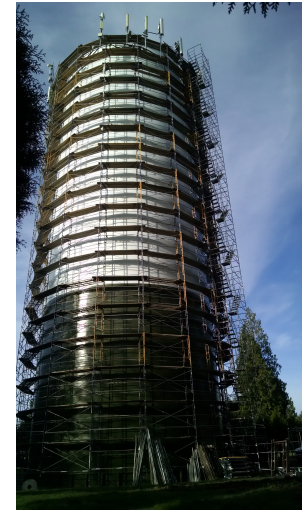
(tank 2 ready for recoating)
