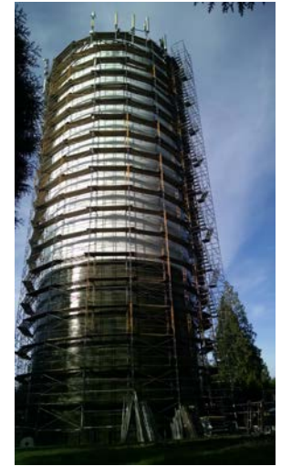
(tank 2 ready for recoating)
